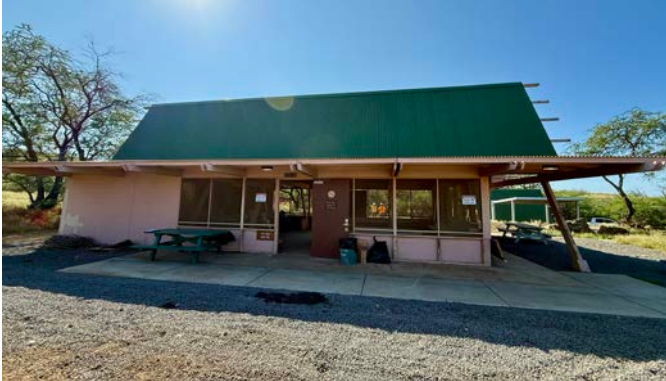
Pavilion at Hapuna State Recreation Area
